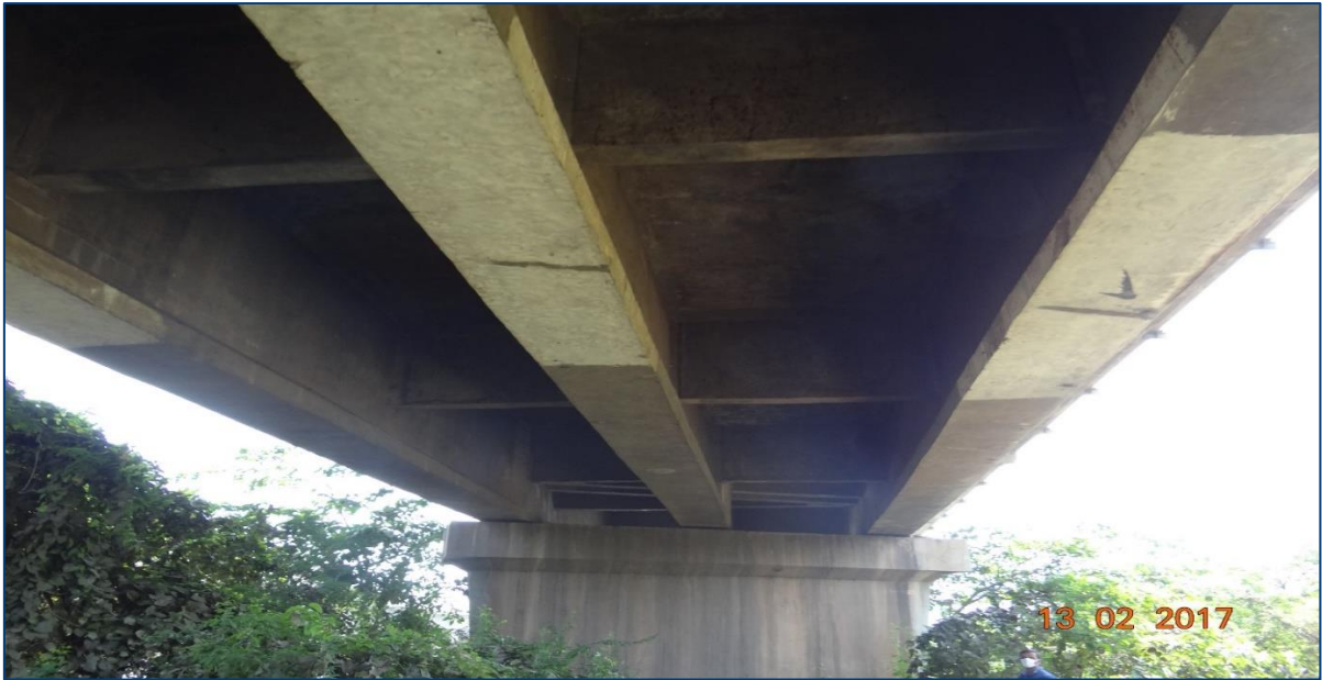
Figure 5: Longitudinal Girders of the bridge.
