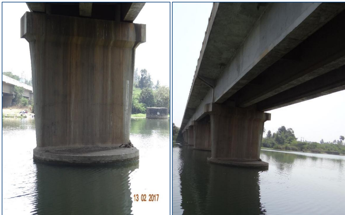
Figure 8: Piers of the bridge submerged in River
