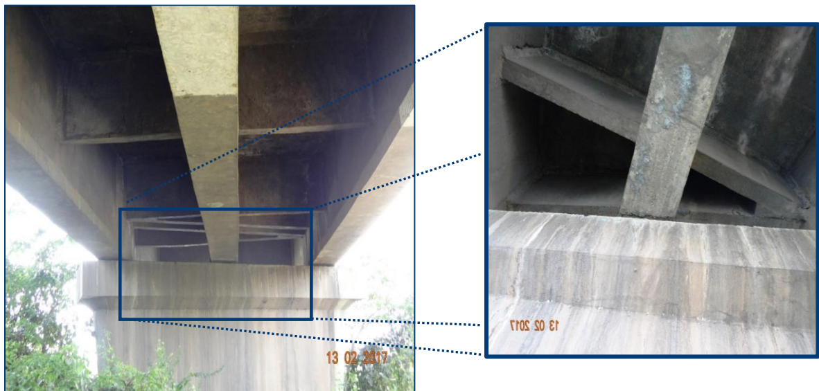
Figure 6: Cross Girders of the bridge.
