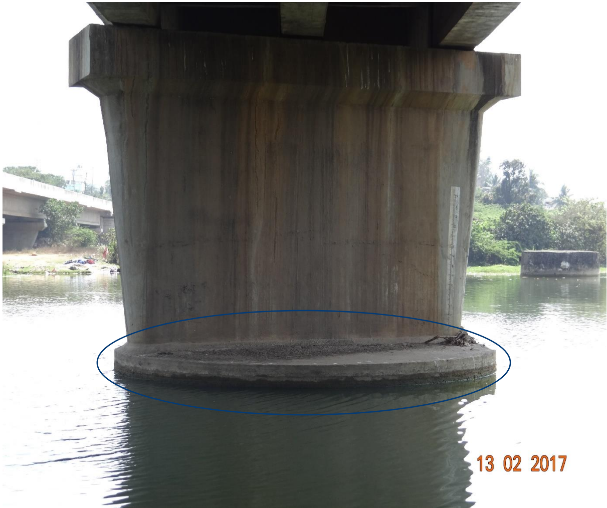
Figure 9: Pile Foundations of the Bridge
