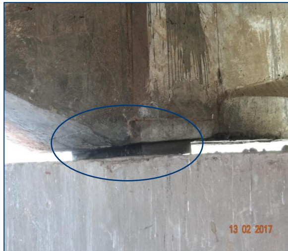
Figure 7: Bearing on Pier showing non-uniform contact.
