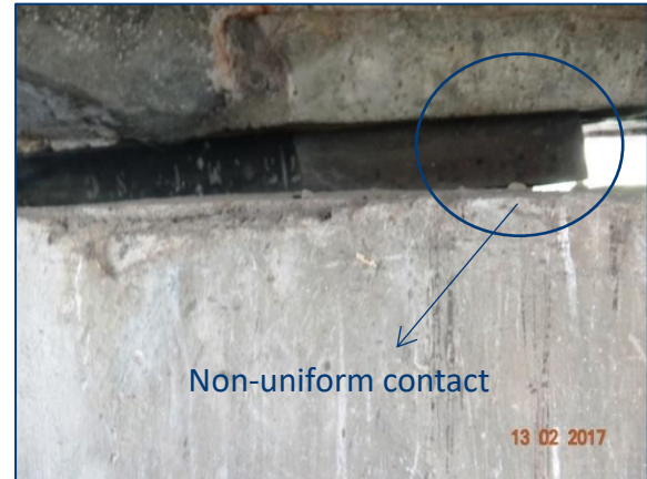
Figure 7: Bearing on Pier showing non-uniform contact.
